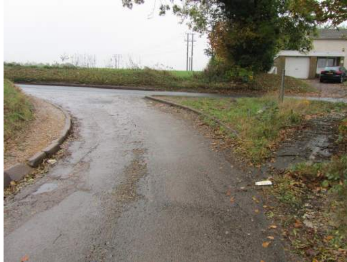
Photograph 18: Buildout to Restrict Turning Movements at Old Lane / Watton Road Junction
