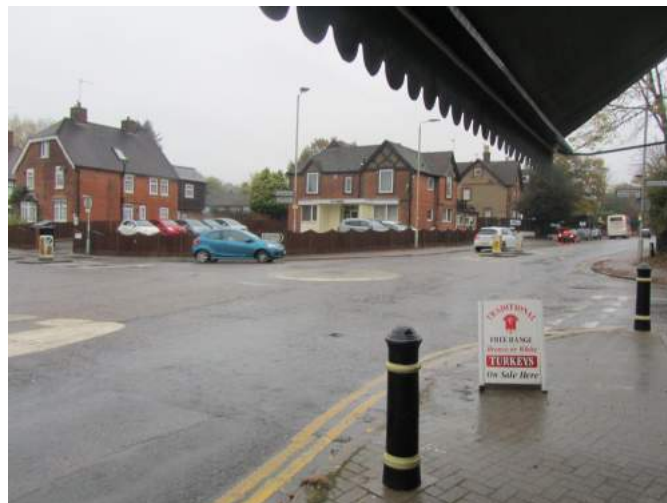
Photograph 1: Existing Mini-roundabout at the London Road / Watton Road Junction
