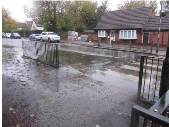
Photograph 7: Standing Water at the Zebra Crossing on London Road
